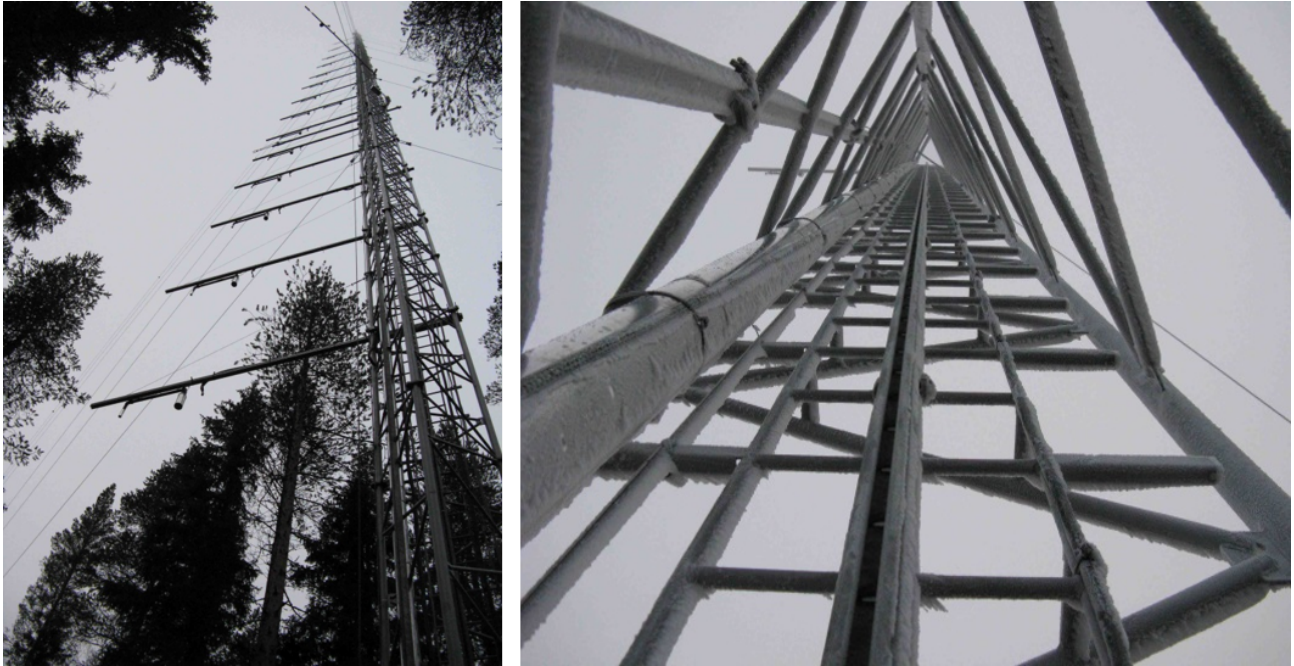
Figure 3: Storage system structure at SE-Svb.
