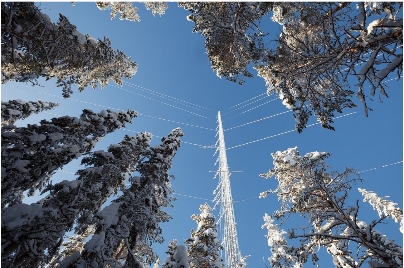
Figure 1 - The SE-Svb tower
