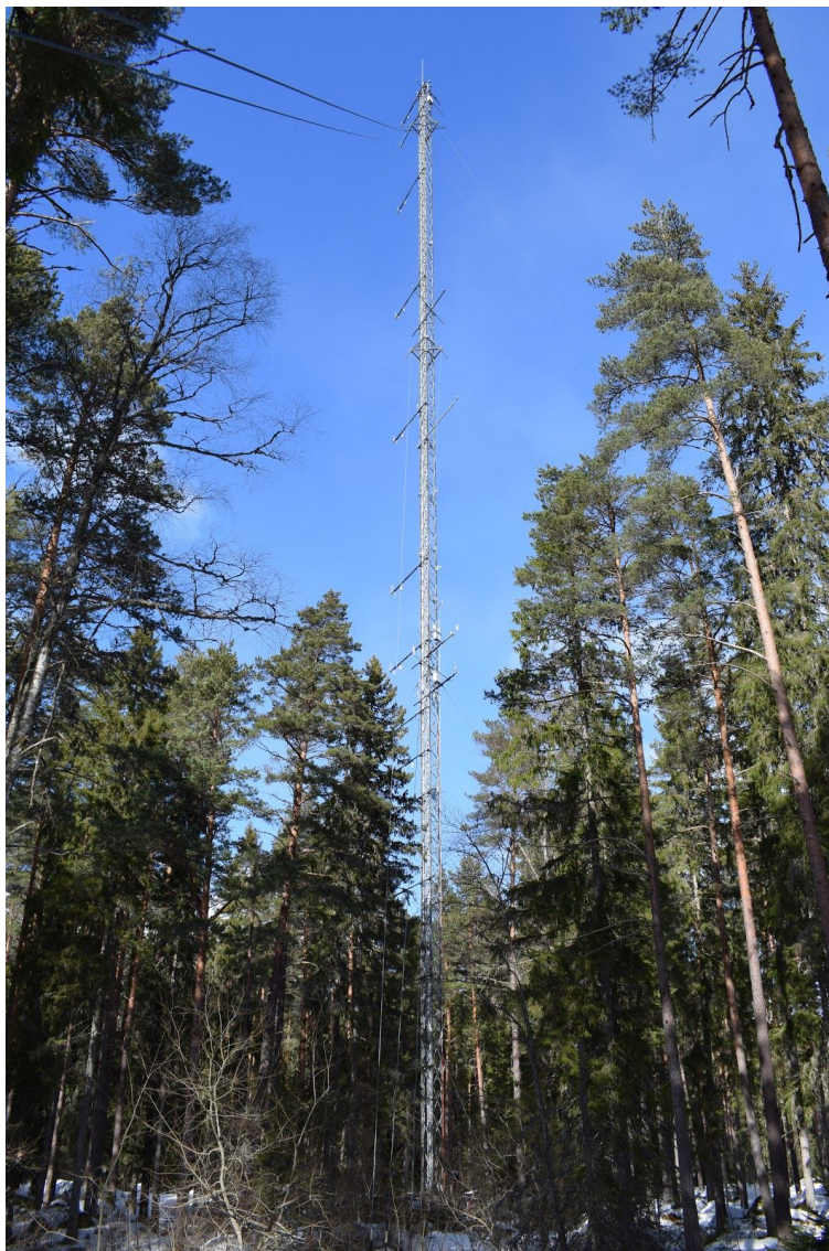
Figure 1 - The SE-Nor tower
